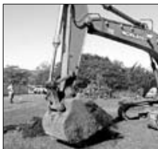
Construction begins on the new pool.
